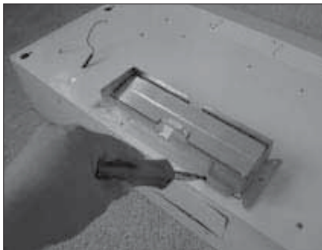
5. Secure 3-1/4" x 10" starting collar with damper to the duct opening using (10) M4x8 screws.
